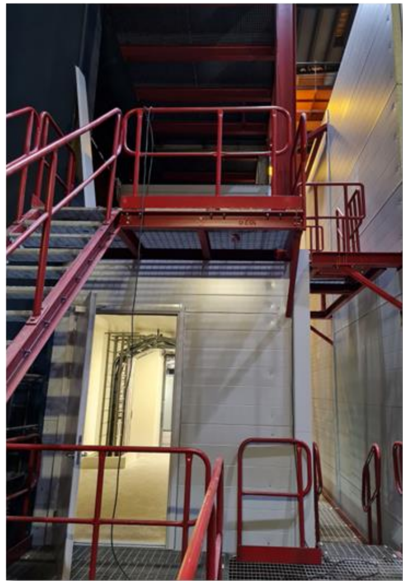
Utility rooms installation
