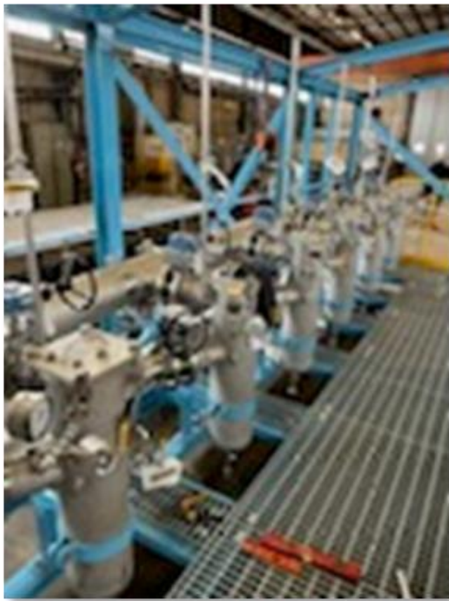
BOFG filtration & sampling station and pipeline
