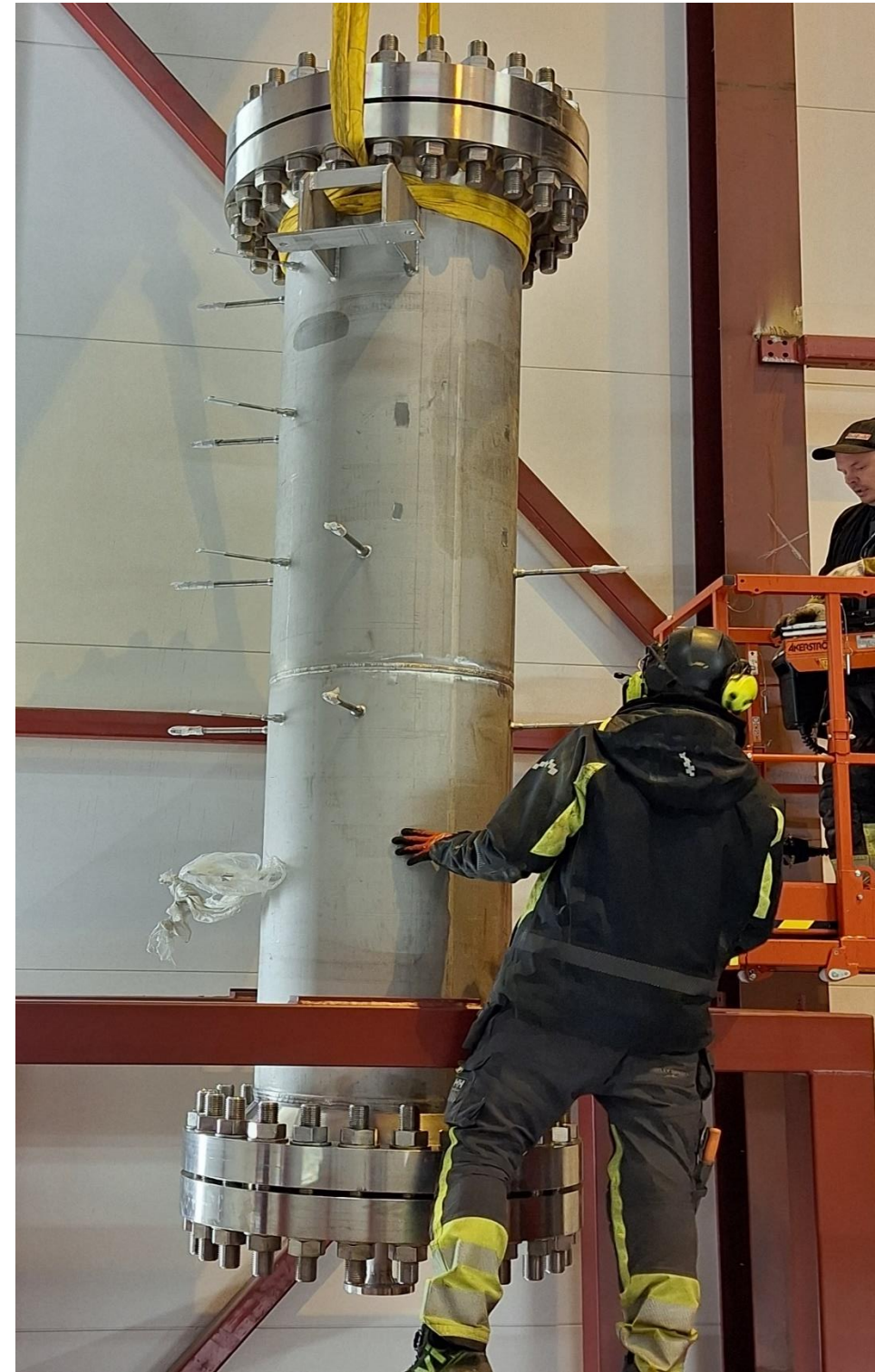
Hoisting the WGS reactor into place
