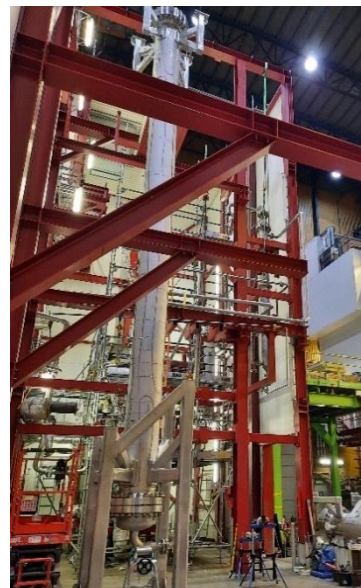
Figure 3: pilot under construction
