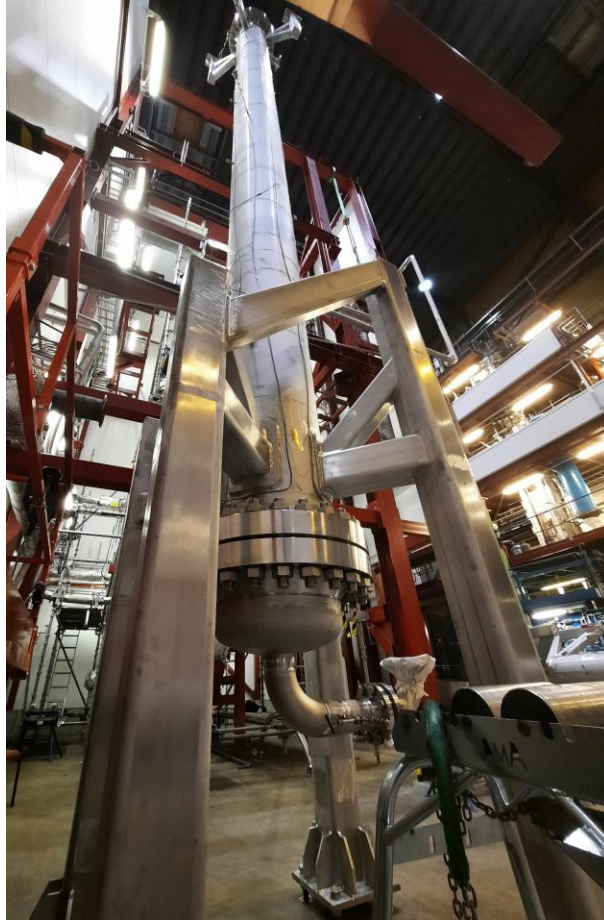
Hoisting the WGS reactor into place
