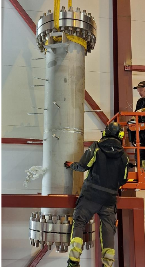
Hoisting the WGS reactor into place
